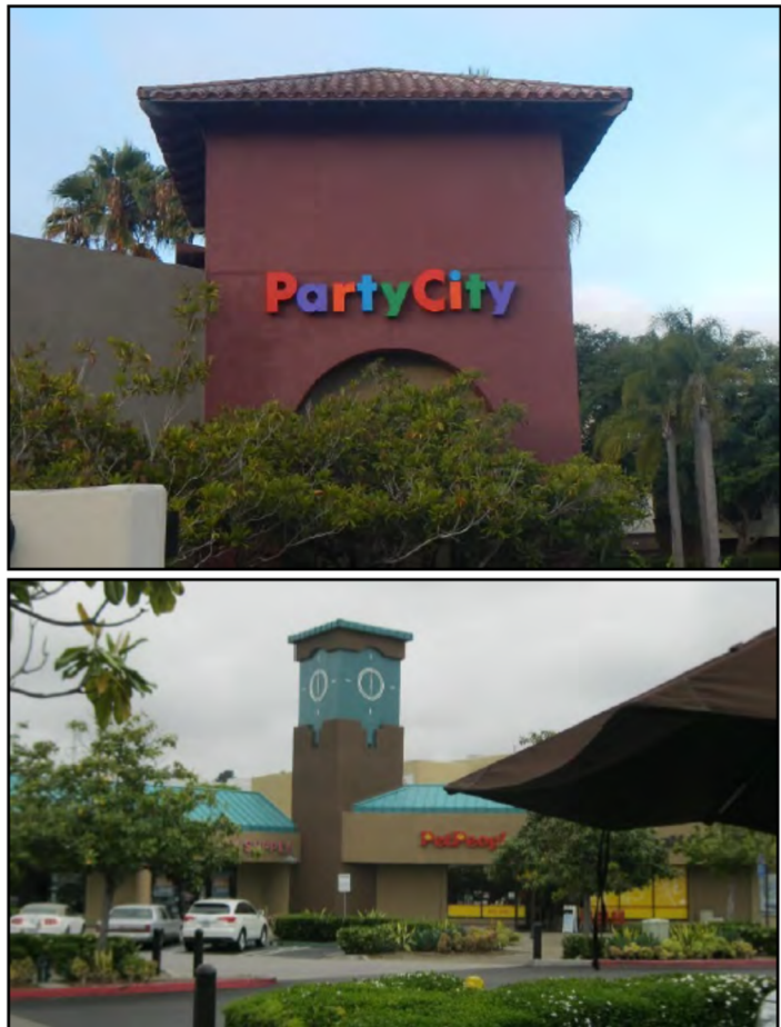
Figure 4: A cupola (above) and a clock tower (below) conceal antennas.
