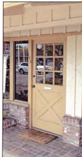
A wood door and brick paving contribute to this inviting shop entry.
