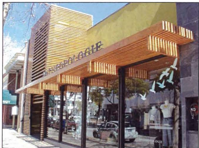
The warmth of the materials and the variety of smaller scale detailing help this modern facade to fit into a streetscape of diverse architecture.
