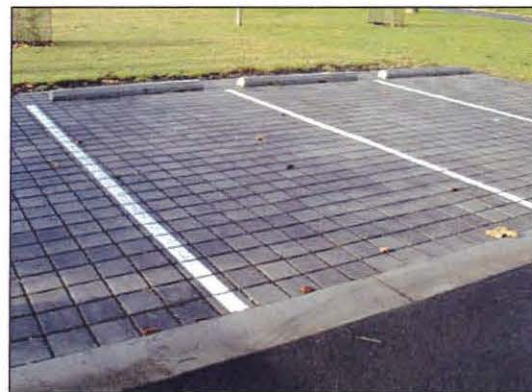
Another example of porous paving
