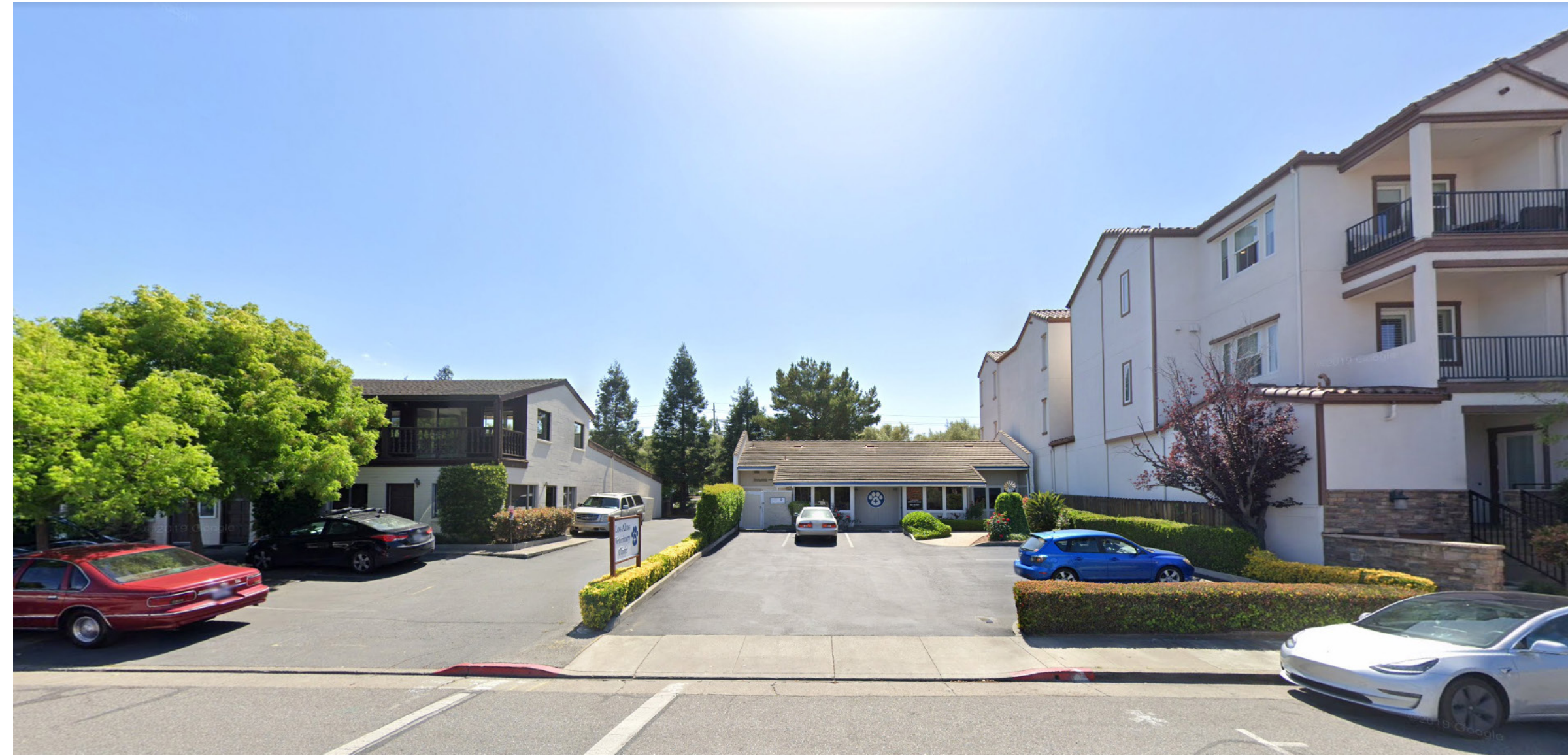
5. Facing the Project on First St
