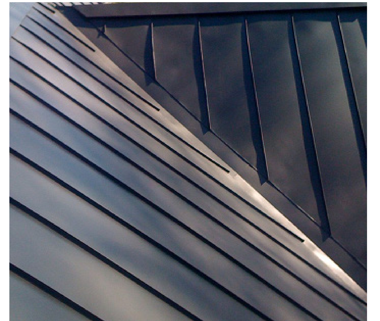
Metal Standing Seam Roof - Dark Bronze Finish
