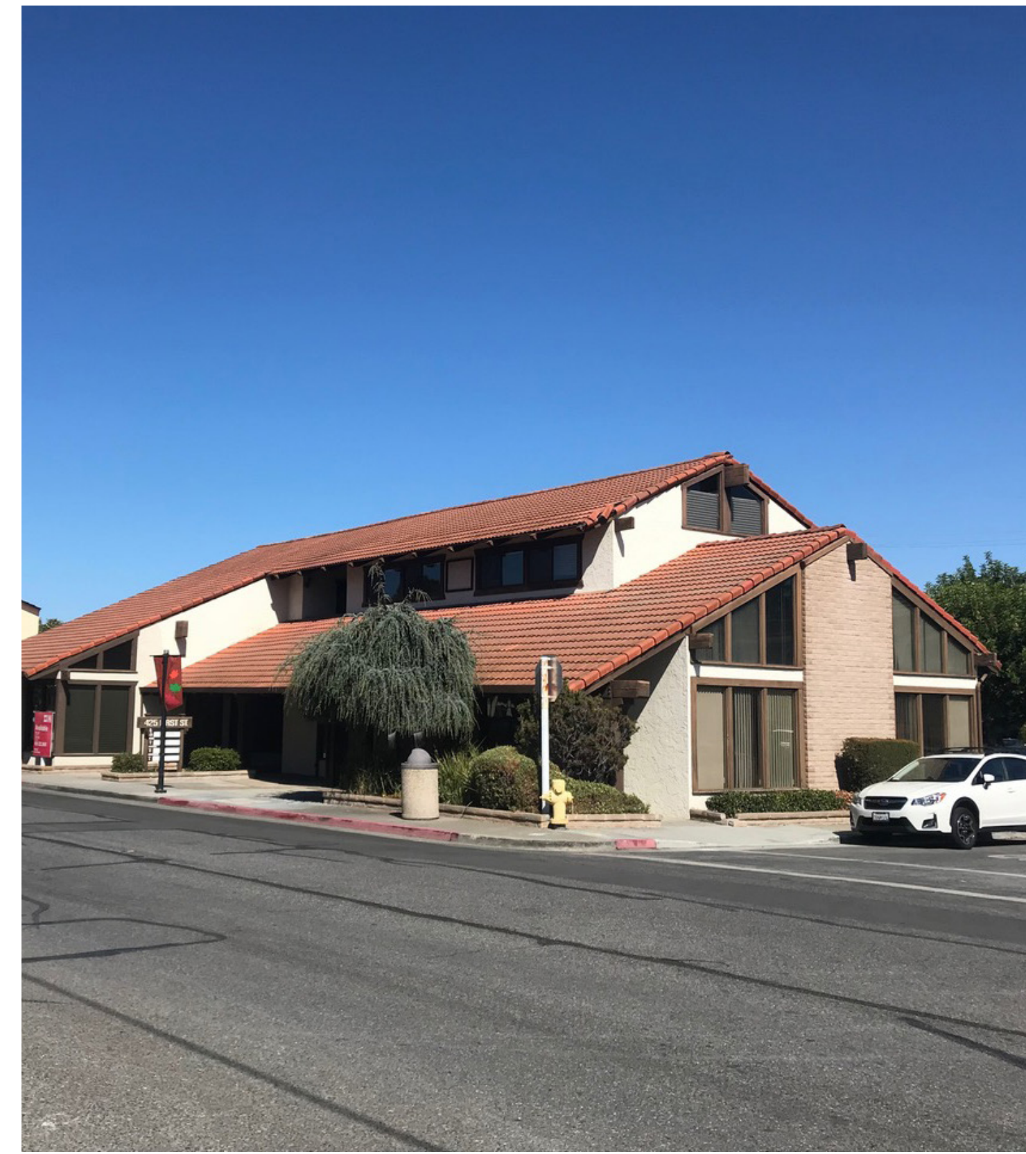
3. Existing Bldg across First St at corner of Lyell
