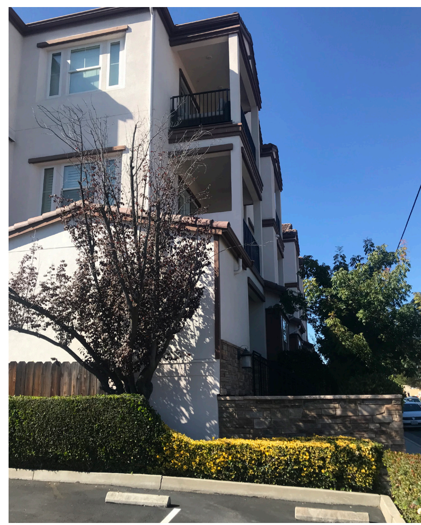
6. First St frontage to the North
