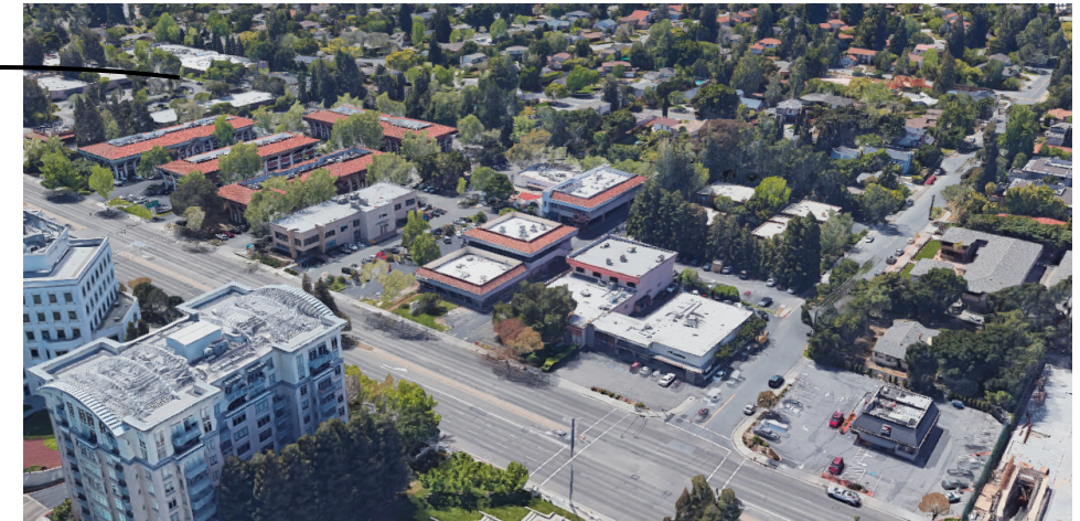
El Camino Real corridor, looking SOUTH near Jordan Ave
