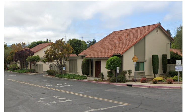
Sweet Oak Street near Homestead Rd
