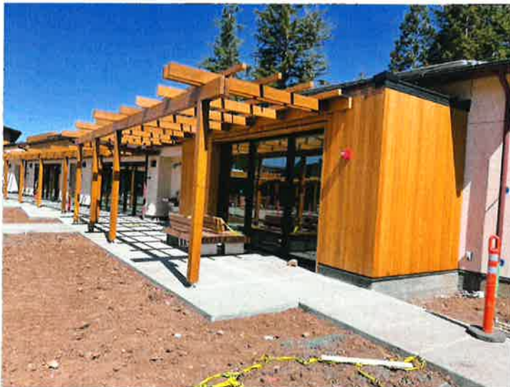
Exterior Progress at Courtyard
