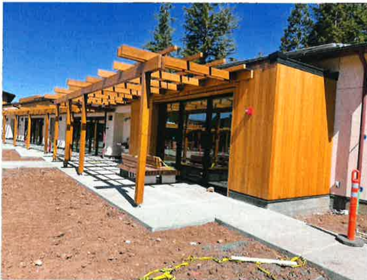
Exterior Progress at Courtyard
