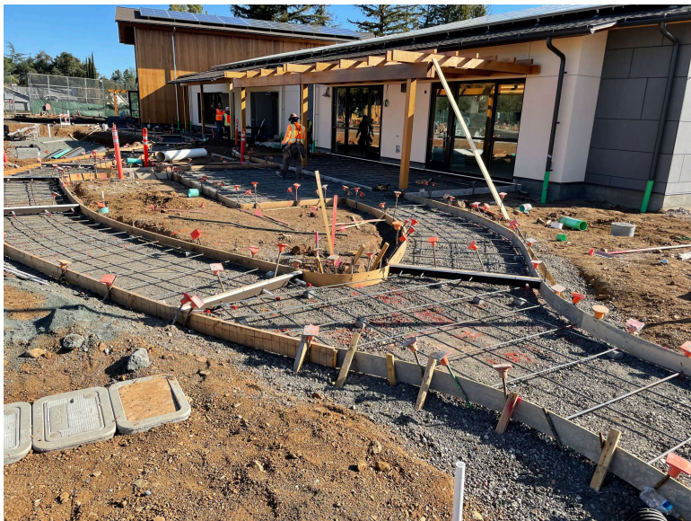
Exterior Progress at Western Site
