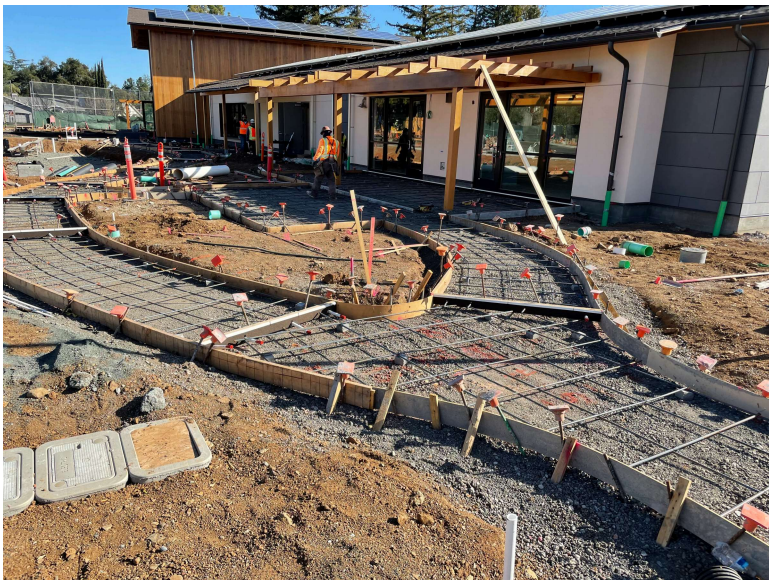
Exterior Progress at Western Site
