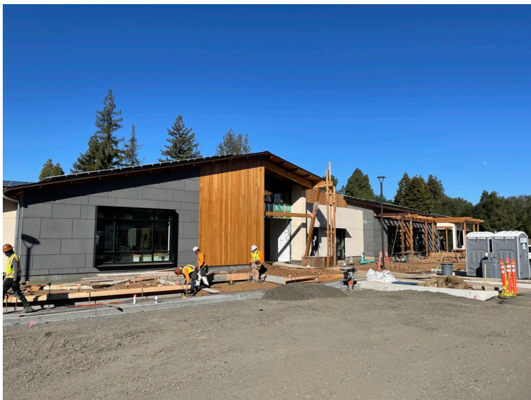
Exterior Progress at South Entrance
