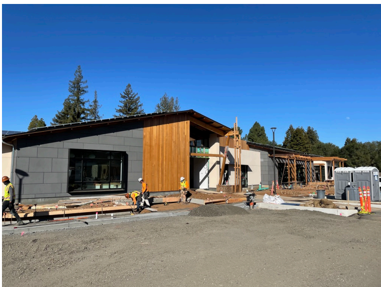
Exterior Progress at South Entrance
