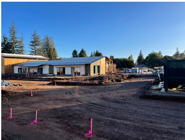
Exterior Progress at South-West Sitework
