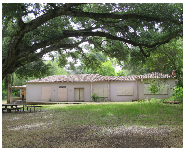
Figure 5. North elevation, 1929 addition at right (photo: ARG, May 2019).
