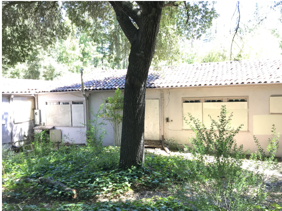
Photo #3 - North End of the West Elevation of the West Wing of the Building
