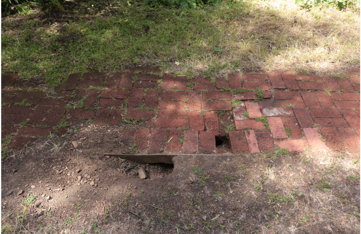
View of walkway paving along east elevation.
