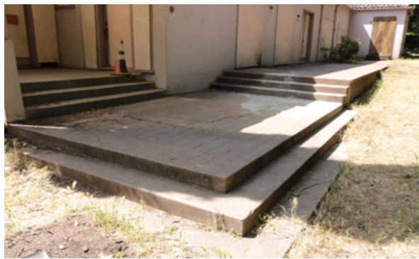
Figure 4. Concrete porch and terrace (photo: ARG, May 2019).
