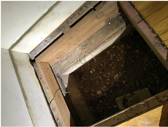
Photo #15: Crawl Space Access Opening in Floor Framing at East Wing
