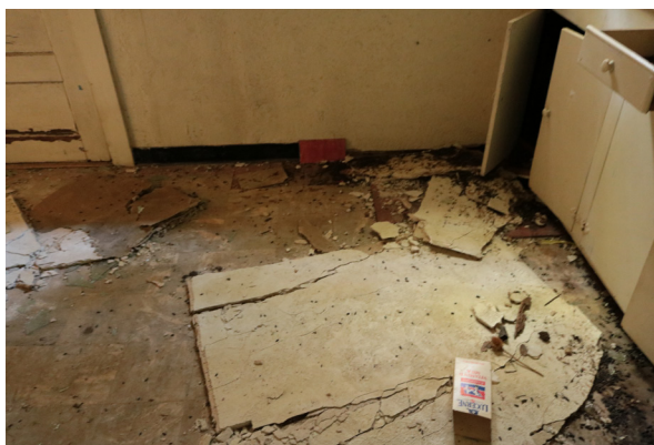
Vinyl tile in the West Kitchen (ARG, 2019).
