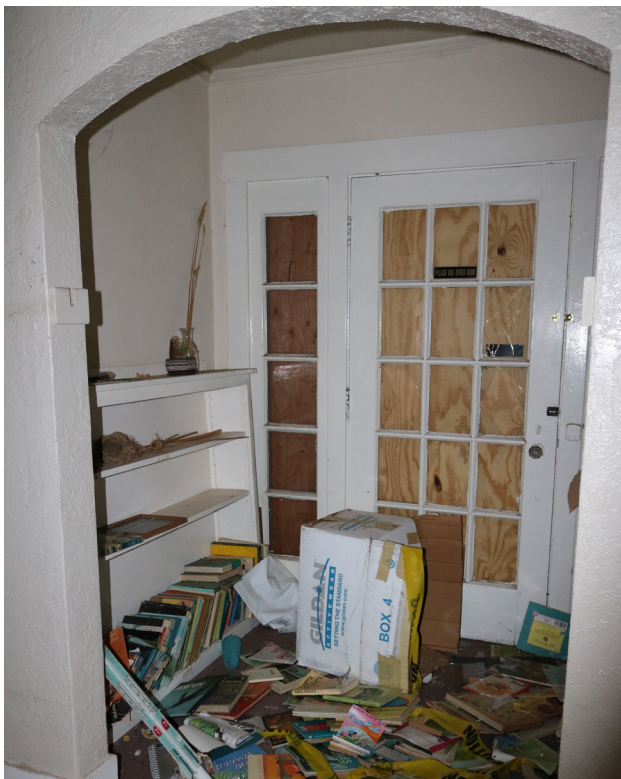
View inside niche at east wall of main room, looking east toward entry.
