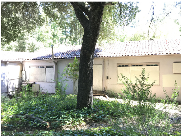
Photo #3 - North End of the West Elevation of the West Wing of the Building
