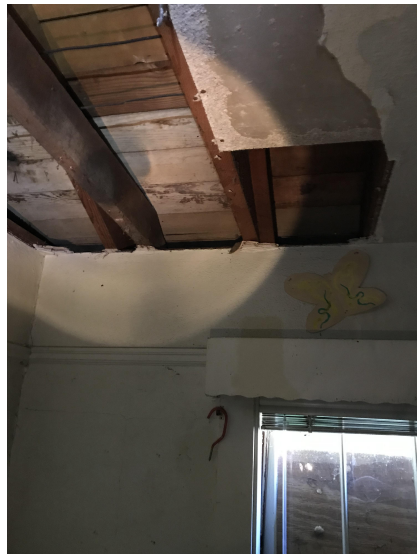
Photo #14: Roof Framing and Ceiling Joist at East Wing of the Building
