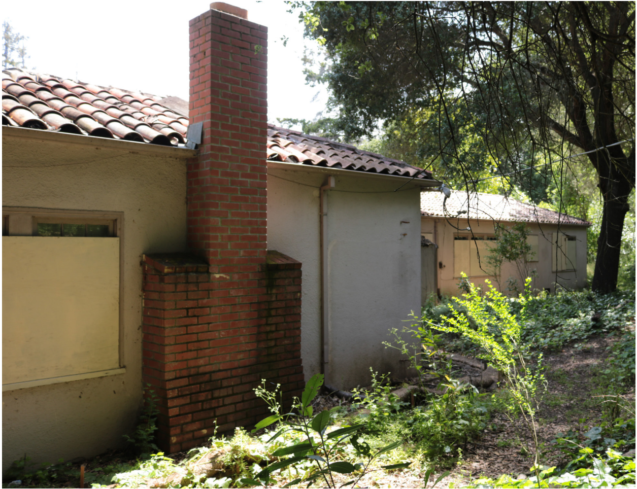
Looking south along the west elevation.
