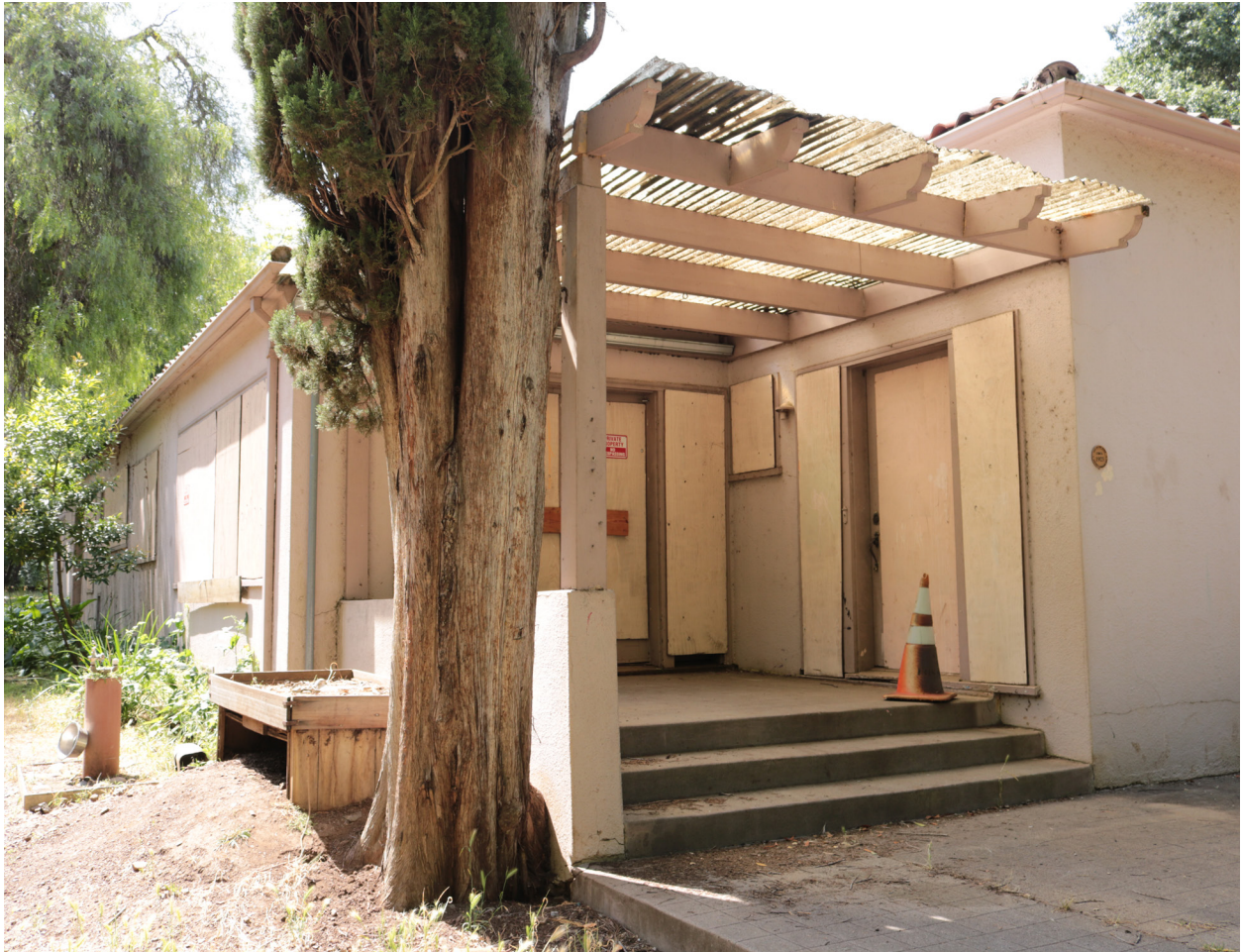
View of northeast corner of Halsey House, including main entrance.
