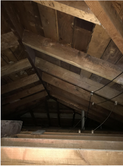
Photo #11: Roof Framing and Ridge Board at West Wing of the Building
