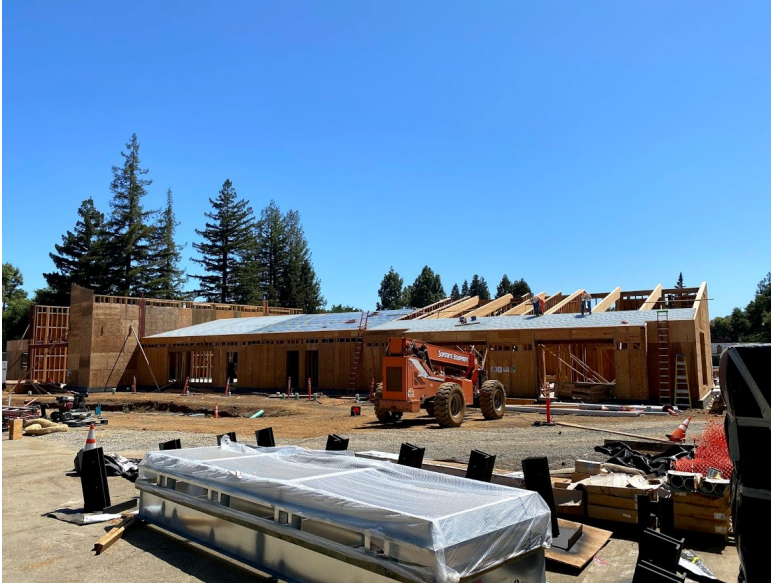
Continued wall and roof framing
