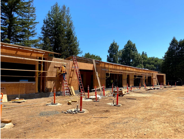
Eave and rafter tail framing at North side of building
