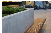
CANTILEVERED WOOD BENCH & PLANTER RETAINING WALL
