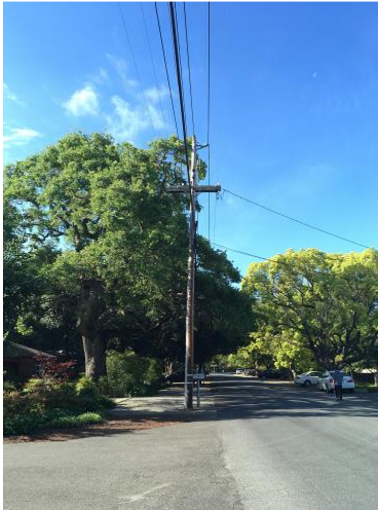
Photo of Existing Pole
