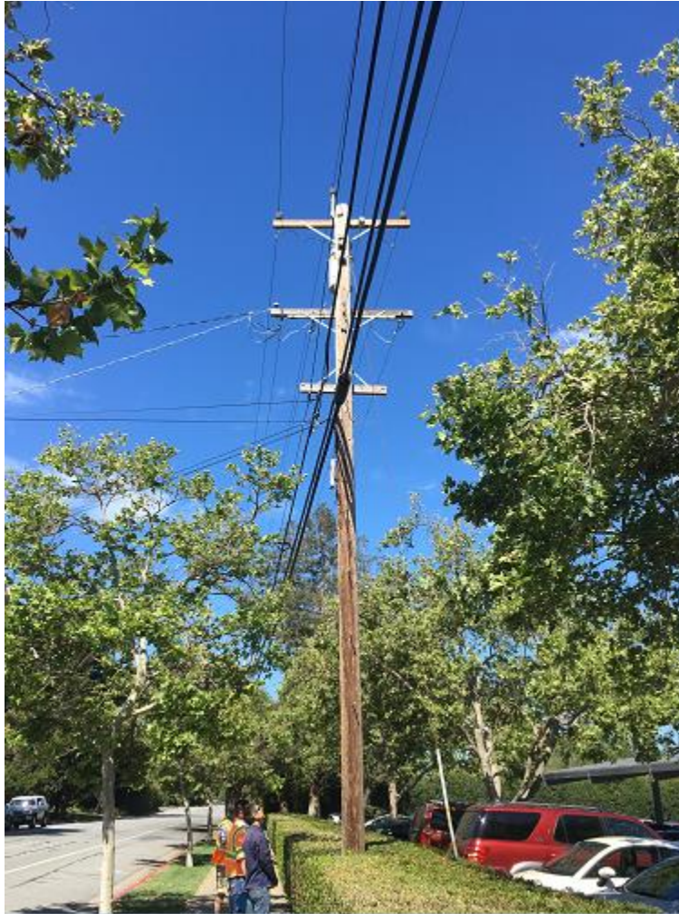
Photo of Existing Pole
