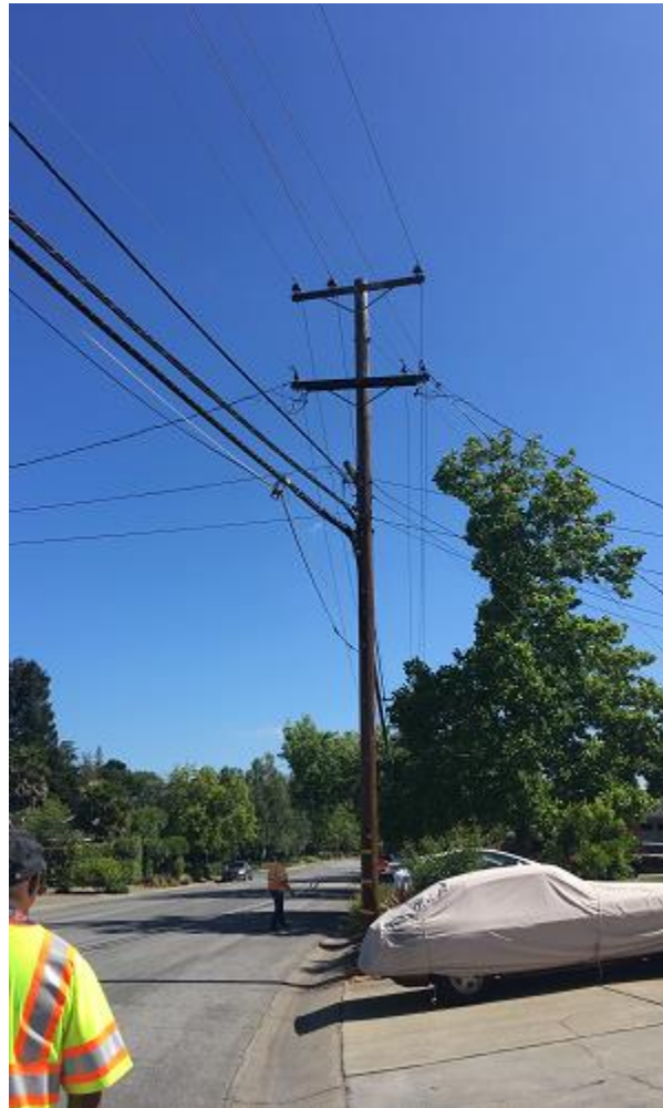
Photo of Existing Pole
