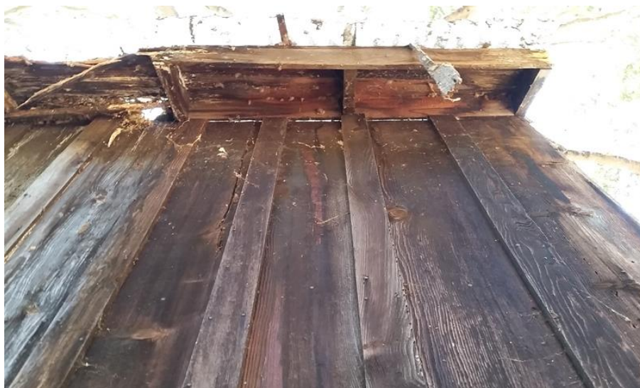
Detail of Eaves – West Elevation, viewed facing east. (July 2016)
