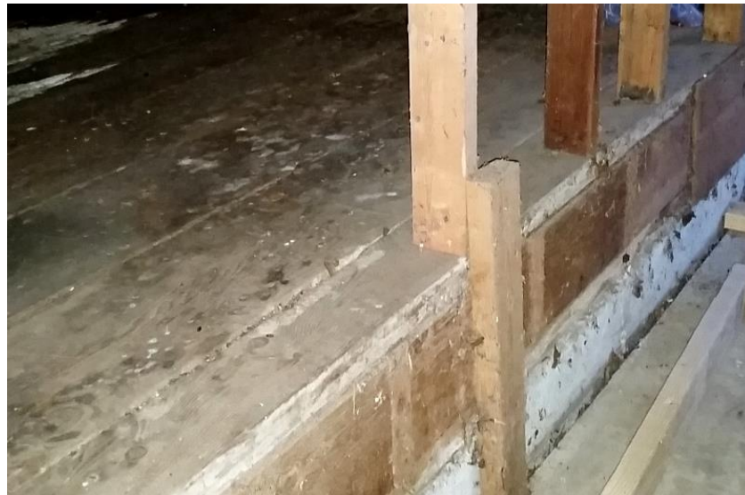
First Floor Raised Floor Framing, viewed facing northwest. (July 2016)
