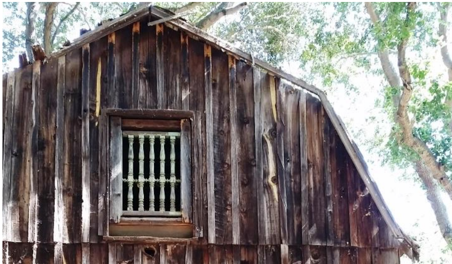
Detail of Gambrel End – South Elevation, viewed facing north. (July 2016)
