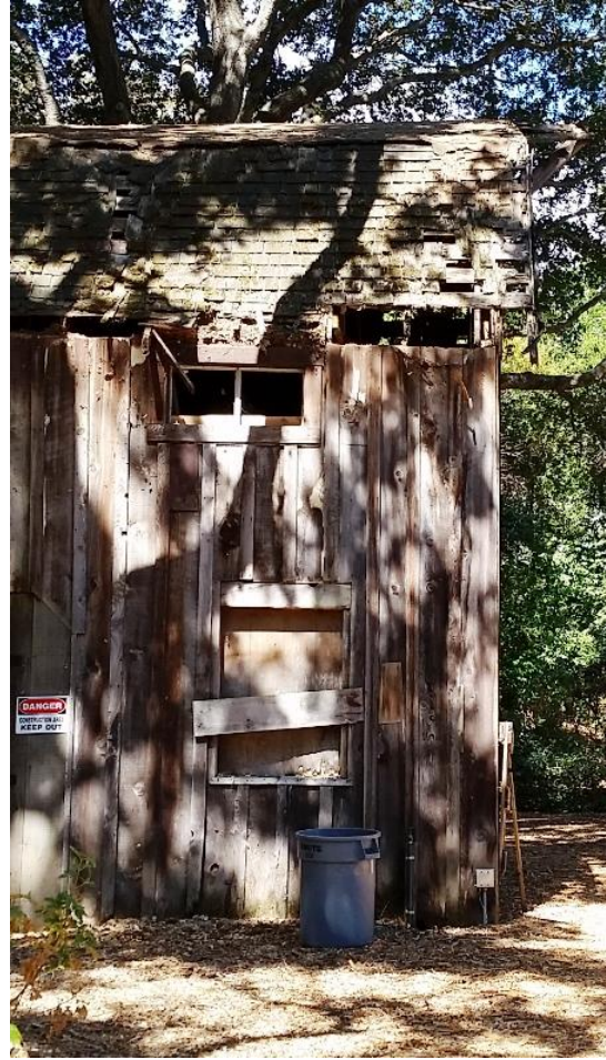
Detail of Northeast Wall, viewed facing west. (July 2016)
