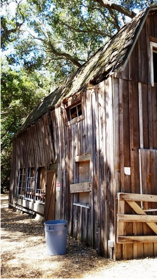
East Elevation, viewed facing south. (July 2016)
