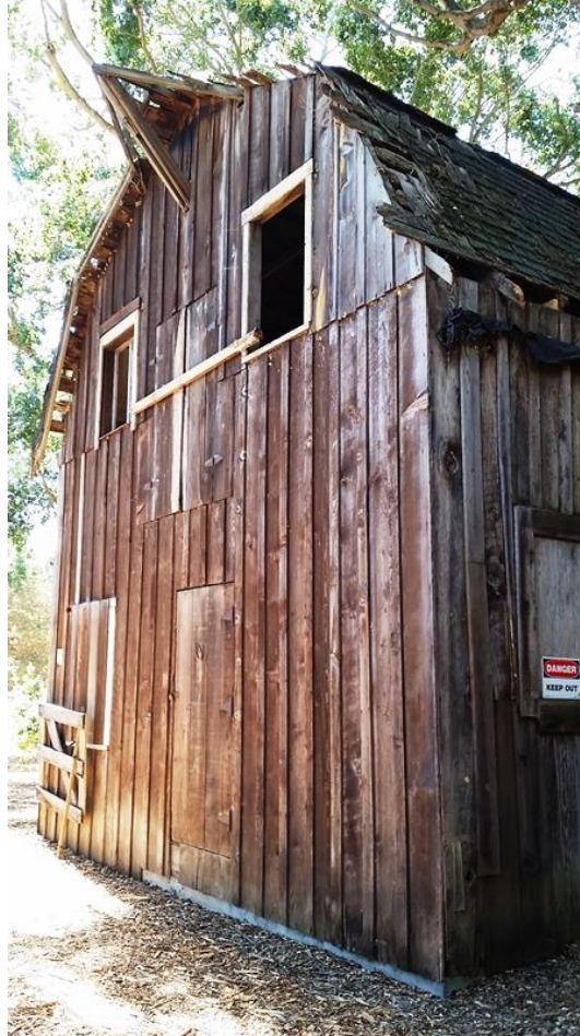
North Elevation, viewed facing southeast. (July 2016)
