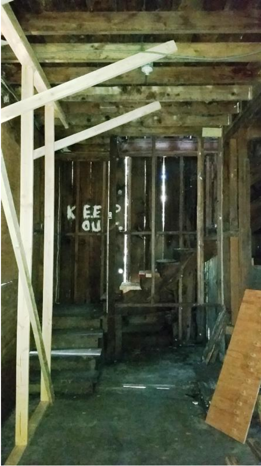
First Floor Interior, viewed facing south. (July 2016)
