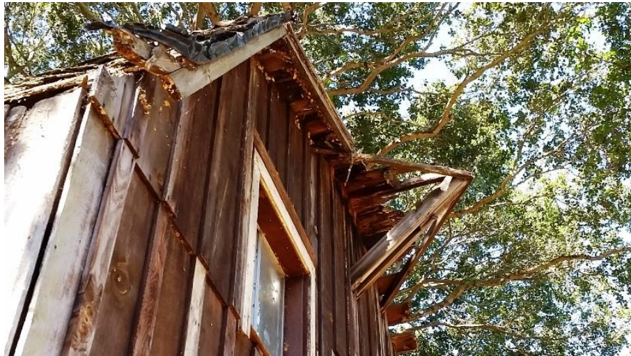
Hay Hood Detail – North Elevation, viewed facing west. (July 2016)
