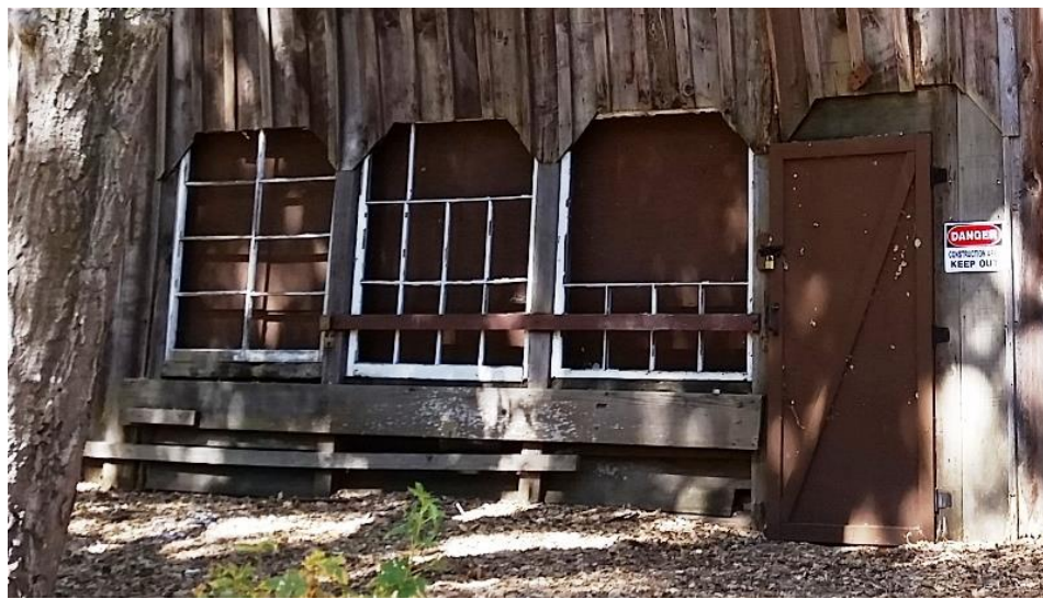
Detail of East Windows, viewed facing west. (July 2016)
