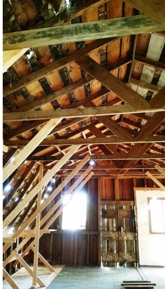
Second Floor Interior, viewed facing north. (July 2016)
