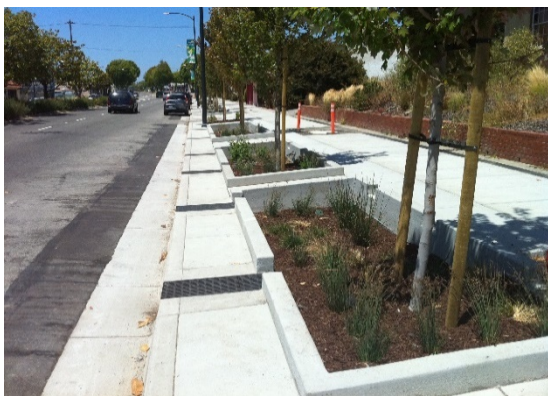
Figure 2-1 Stormwater sidewalk planters along San Pablo Avenue (Source: EOA)
