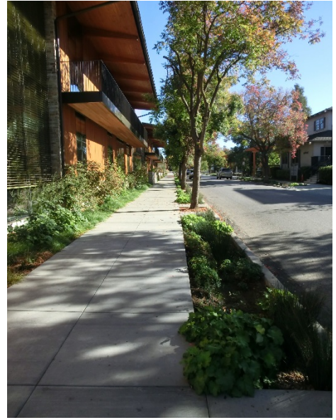
Figure 2-11 David and Lucile Packard Foundation curbside flow-through rain garden (Source: EOA, Inc.)
