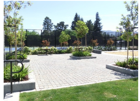
Figure 2-4 Plaza with permeable pavers, Rosita Park (Source: City of Los Altos)
