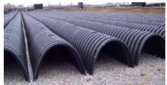
Figure 2-6 Subsurface infiltration system (Source: Contech)
