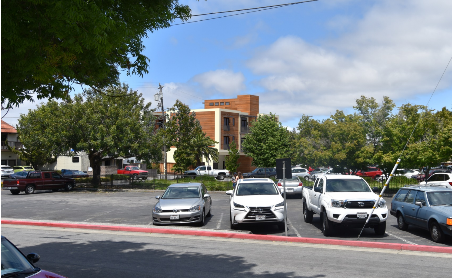
VIEW FROM SECOND STREET & LYELL STREET
