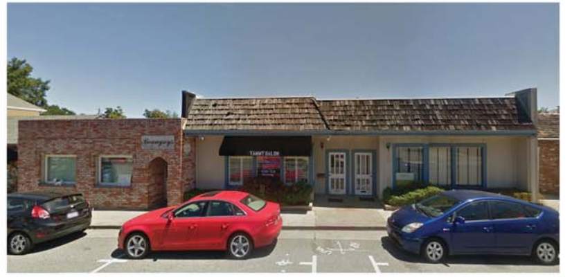
389 FIRST STREET - EXISTING SITE
