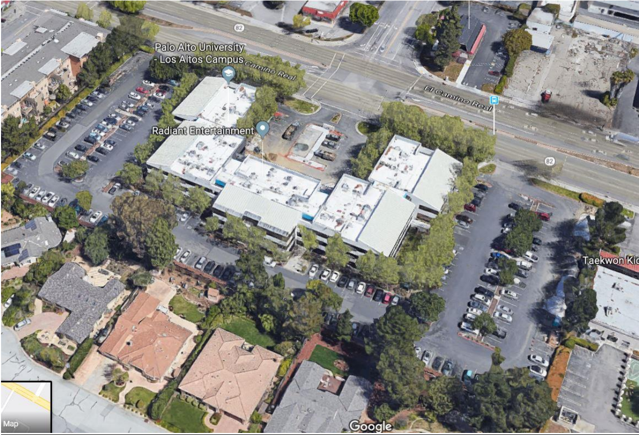
Aerial view of 5150 El Camino Real existing conditions including parking lot uses
