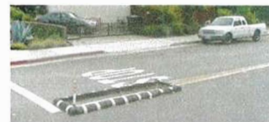
Figure 3 – Example of a Narrow Median Island
