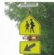
Figure 5 – Example of an (RRFB)
