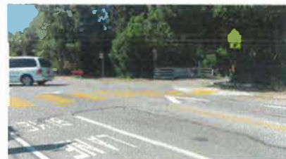
Figure 4 – Example of a Raised Crosswalk
