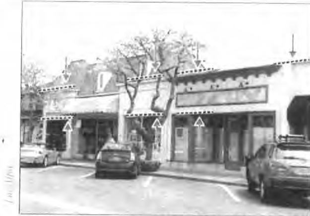
Matching parapet and window heights help relate these adjacent buildings.
