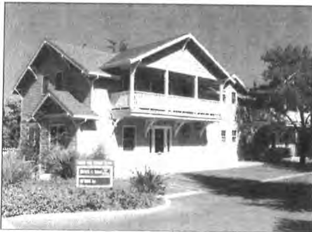
Another example of second floor balcony and deck space providing facade depth and visual interest.
