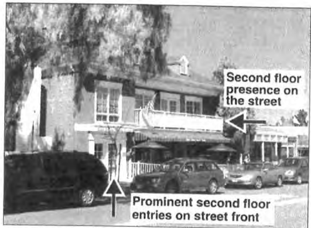
Strong presence of second floor uses on the street
