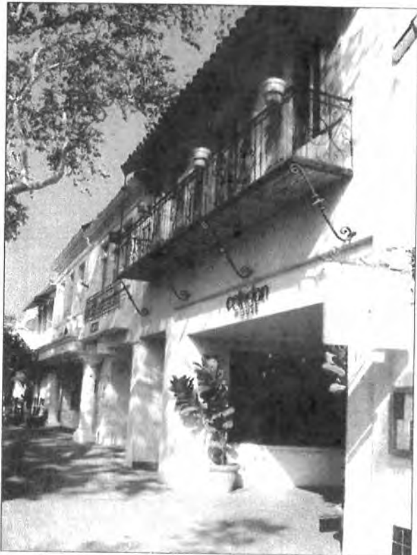
Reinforcing the module with second floor projections and details.
