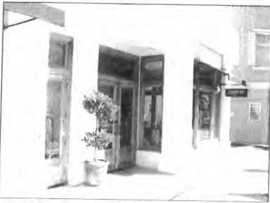
Front facades are predominantly display windows and entries.
