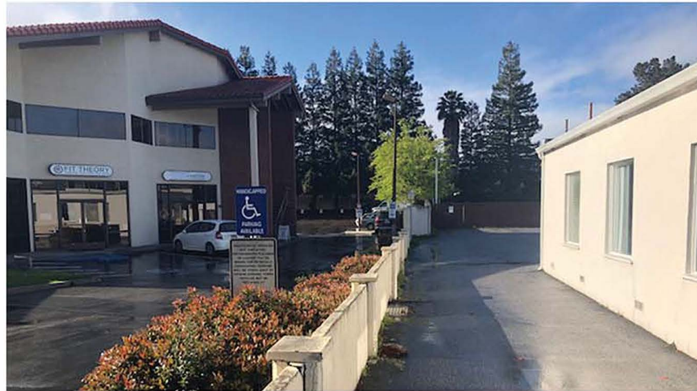
VIEW TOWARDS REAR PROPERTY LINE
