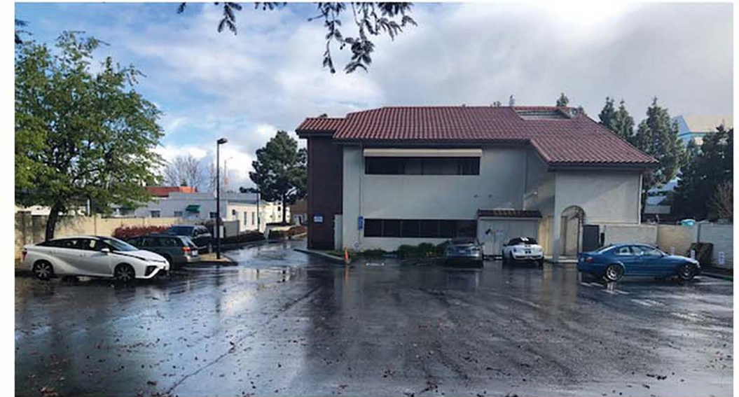
VIEW FROM REAR PROPERTY LINE
