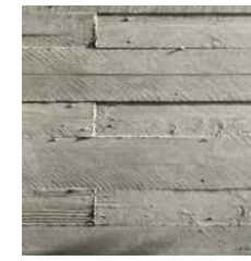
BOARD FORM FINISH CONCRETE
