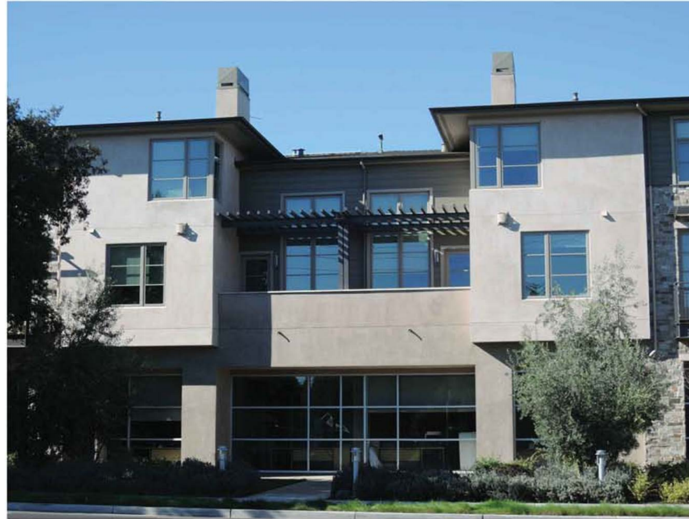
960 NORTH SAN ANTONIO ROAD
