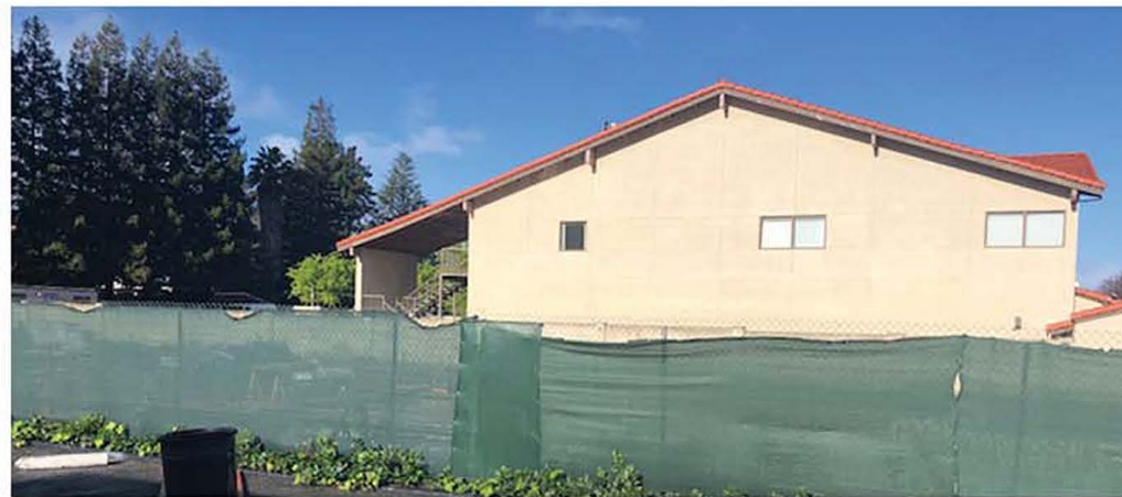
VIEW FROM SOUTHEAST (JACK-IN-THE-BOX)
