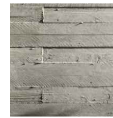
BOARD FORM FINISH CONCRETE
