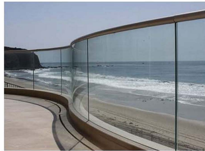
DECK MOUNTED GLASS GAURD RAILINGS
