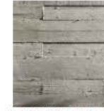
BOARD FORM FINISH CONCRETE
