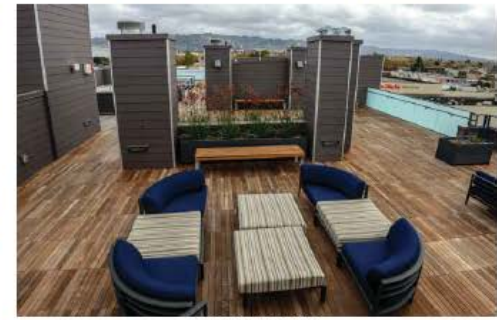
ROOF DECK - WOOD PAVING
