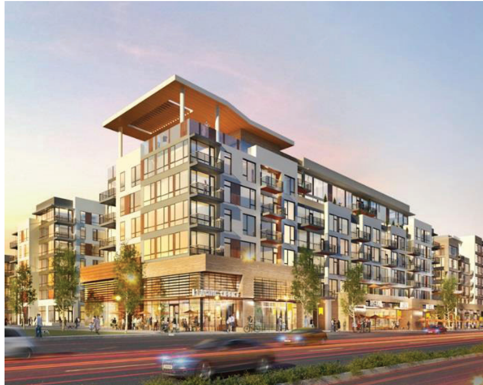
400 SAN ANTONIO RD, MOUNTAIN VIEW (APARTMENT) - APPROVED/ UNDER CONSTRUCTION
