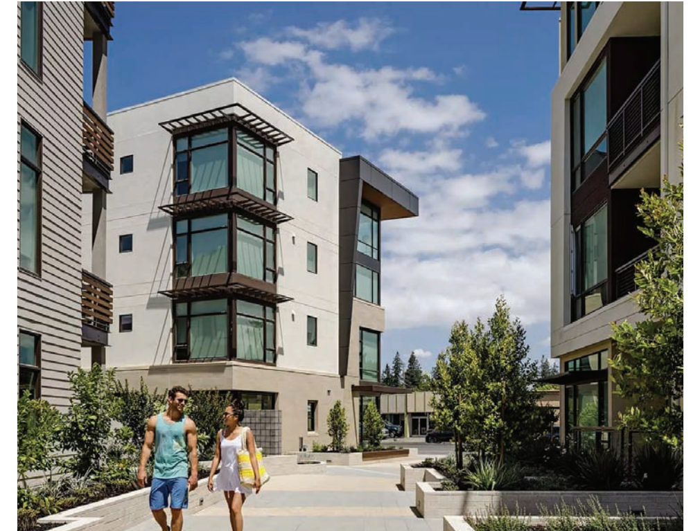
100 MOFFETT, MOUNTAIN VIEW (APARTMENT) - COMPLETED
