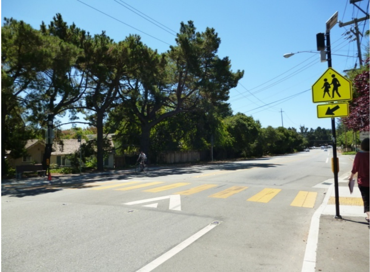
Figure 3-13: A crossing on Grant Road at Morton Avenue includes a raised crosswalk, high-visibility striping, and pedestrian-activated in-pavement flashing lights. St. Simon Elementary School is located on the west side of the crossing. A VTA Route 51 bus stop is to the east.
