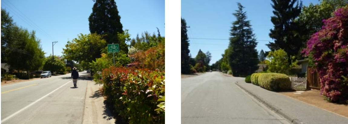
Figure 3-10: Paved shoulders often double as parking lanes, sidewalks, and bicycle facilities in many residential neighborhoods in Los Altos(left). An asphalt berm (right) converts a paved shoulder into an informal walkway.
