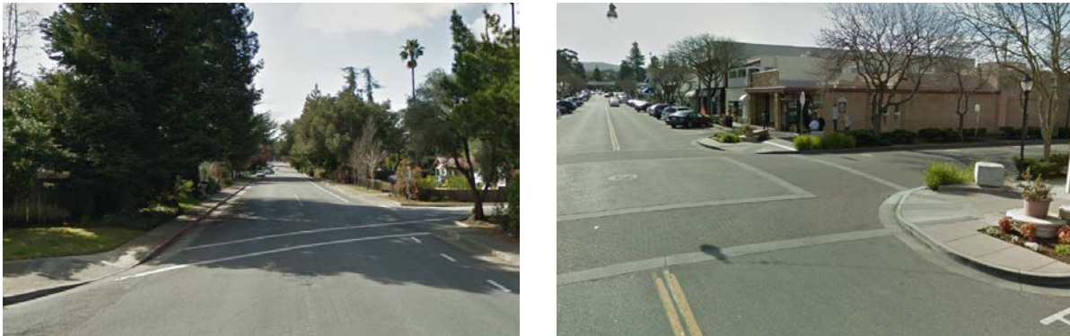
Figure 3-15: Example of a minimal crosswalk treatment across Edith Avenue at 4th Street (left), and a decorative crosswalk with curb extensions on Main Street in downtown Los Altos (right)
