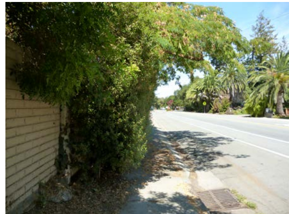
Figure 3-6: Overgrown vegetation on El Monte Avenue
