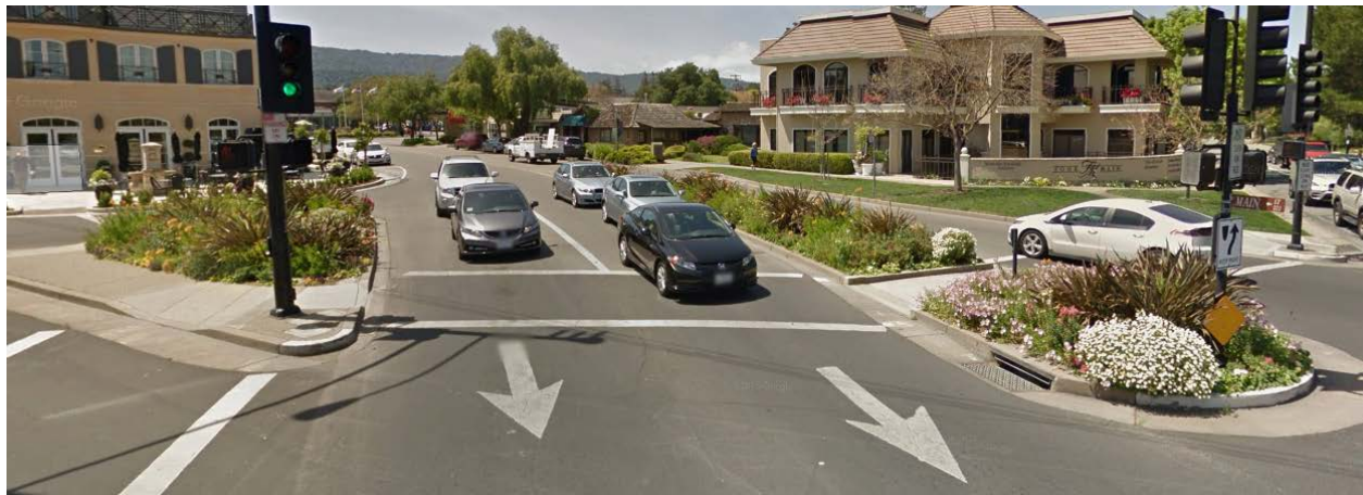
Figure 3-17: Two types of medians—slip lane and center—shorten crossing distances and create a gateway at the skewed intersection of Main Street and San Antonio Road. (Image: Google)
