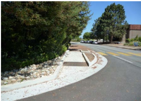
Figure 3-12: Recent improvements across from Blach Elementary School create a protected waiting area and shorten the crossing distance for pedestrians.
