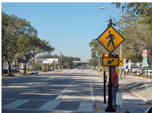
Figure 5-7: Rectangular rapid flashing beacon
