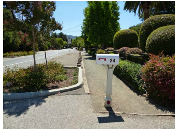
Figure 4-9: A mailbox blocks part of the walkway on El Monte Road
