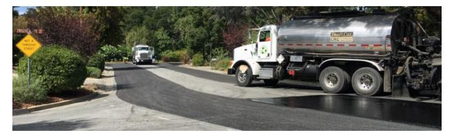
This project slurry seals City streets annually, including cutout and repair of minor pavement failures, and installation of striping. The seal typically places a thin layer of sand and oil over City streets. Neighborhood streets should receive a surface treatment (slurry seal) other than an overlay every seven years. Sealing is a preventative maintenance treatment that prevents moisture from penetrating the pavement and softening the base material supporting the pavement.
