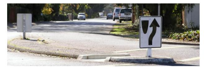
The Intersection Access Barrier Removal project is used to remove barriers that impact accessibility to sidewalks or trails. Typical improvements include reconfiguration of rolled curbs to provide a smooth transition from the street to adjacent pedestrian pathways, removal or reconfiguration of bollards, or reconfiguration of trail entry points to better accommodate bicycle access.
