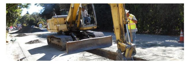
The 2013 Sanitary Sewer Master Plan Update recommended replacement of segments of pipes located at various locations throughout the City that are included in the 30-day focused cleaning schedule that have severe sags. Such sags can cause accumulation of debris and grease which necessitates frequent cleaning.
