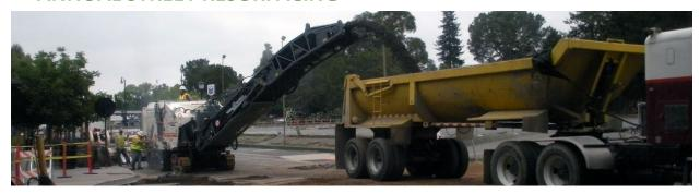
The annual street resurfacing project places an overlay of asphalt concrete (AC) on existing street surfaces that are approaching the end of their useful life, as evidenced by cracking and minor pavement failures. Installation of pavement fabric in addition to pavement striping and stenciling after the resurfacing, repair of damaged curb and gutter, and minor drainage improvements are also included in this project.
