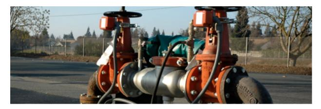
The project will install backflow preventers for all City-metered water connections. The Cross-Connection Control Program is designed to meet the requirements of the California Code of Regulations, Title 17, Public Health Sections 7583 through 7605. Failure to install and maintain such devices may lead to a water service interruption and possible loss of water services.
