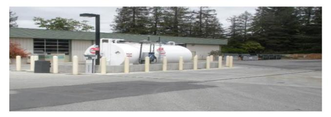
The fuel dispensing island at the Municipal Services Center (MSC) has an above ground holding tank with a containment wall around it. It is necessary to build a canopy to limit storm water from entering the contained area and to provide cover for the fueling station to prevent excessive weathering of the electronic screens and keypads.
