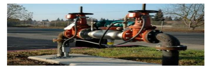
The project will install backflow preventers for all City-metered water connections. The Cross Connection Control Program is designed to meet the requirements of the California Code of Regulations, Title 17, Public Health Sections 7583 through 7605. Failure to install and maintain such devices may lead to a water service interruption and possible loss of water services.
