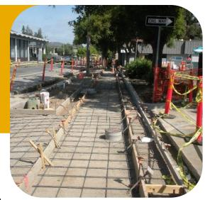
This project provides for replacement of cracked or uplifted sidewalks throughout the City that cannot be patched or ground down.
