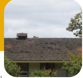
due to the failing materials on top. A complete tear-off of the existing roof is needed, and a new wood shake roof needs to be re-laid along with new felts/tar papers.
