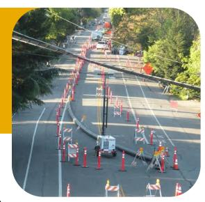
The work is in the largest pipe diameter sections in the system that delivers sewage to the Palo Alto Regional Water Quality Control Plant. The trunk sewer rehabilitation is divided into several phases to be more manageable and provide flexibility to rehabilitate the reaches that are most corroded as determined by future, more in-depth inspections of the trunk sewer pipe.
