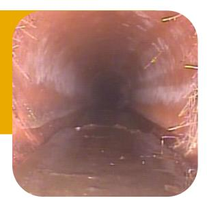
Inspection programs are required to determine current sewer conditions and to aid in planning a maintenance strategy. Video inspections are the most frequently used, most cost efficient, and most effective method to inspect the internal condition of a sewer.
