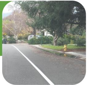
This project will refresh City streets with thermoplastic pavement striping each year. It will also improve striping layouts per the City's Pedestrian Master Plan and Bicycle Transportation Plan where appropriate. Thermoplastic lasts for approximately seven to eight years. This project allows the City to complete a striping cycle on an eight-year basis in accordance with requirements and to maintain the acceptable conditions.
