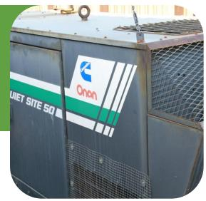
Equipment Registration Program. The generator is subject to unscheduled inspections by the State for compliance with emission requirements. While the existing generator is meeting the current emission requirements, it is aging and at risk of exceeding emission standards soon. The new more energy-efficient Cummings generator will meet all BAAQMD requirements and will be more cost-effective to operate.
