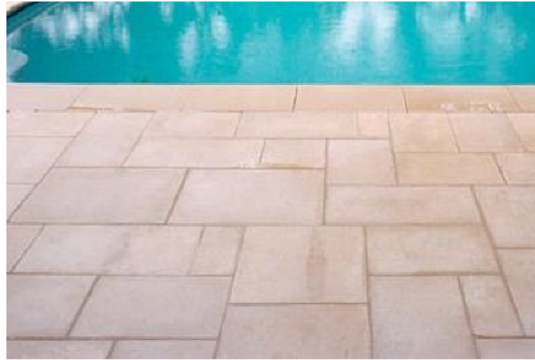
PRECAST CONCRETE PAVING
