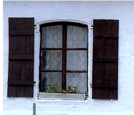
Inset casement windows with bullnose stucco surround
