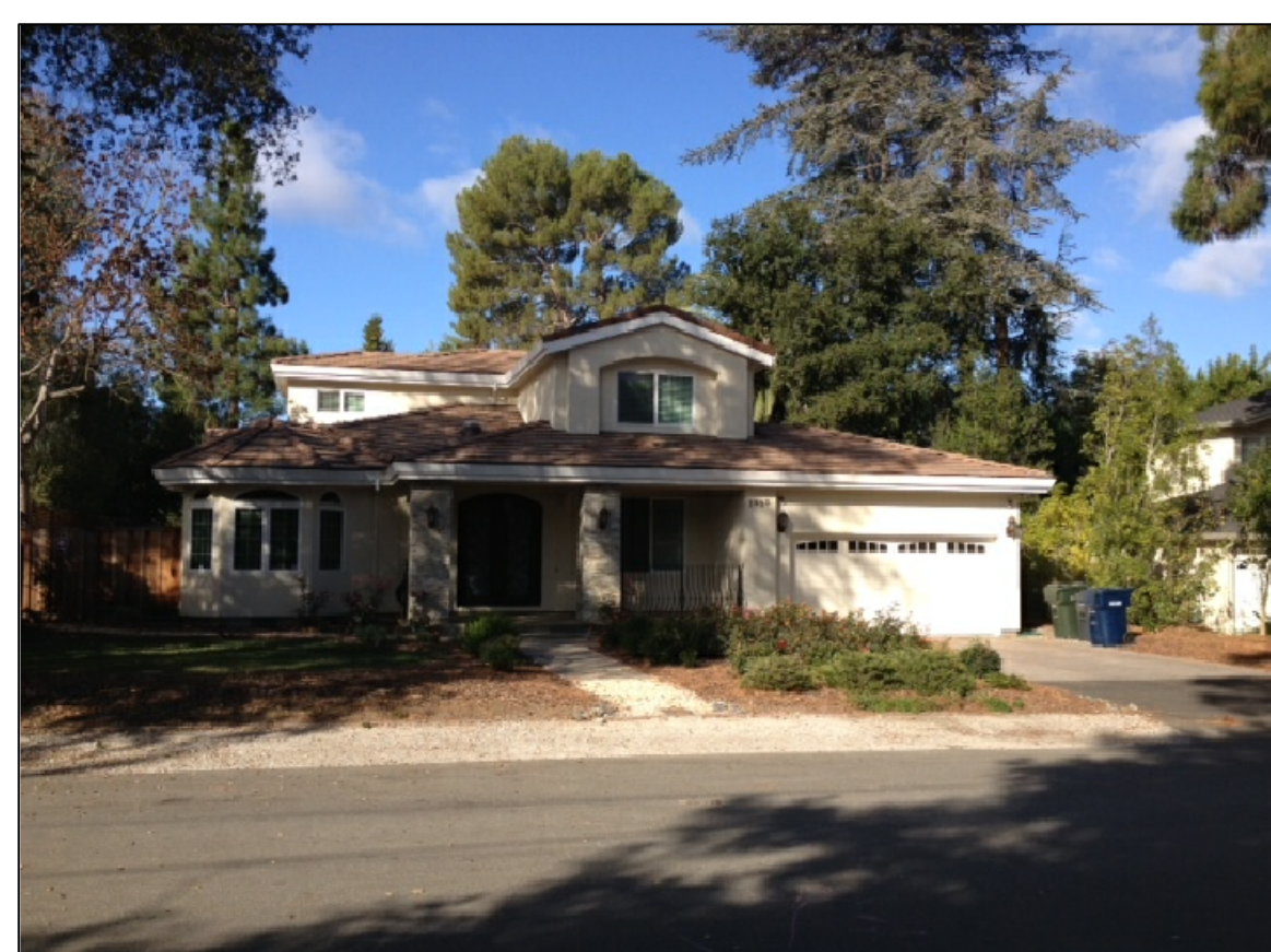
1052 RAY AVE (ACROSS STREET OF PROPOSED RESIDENCE)
