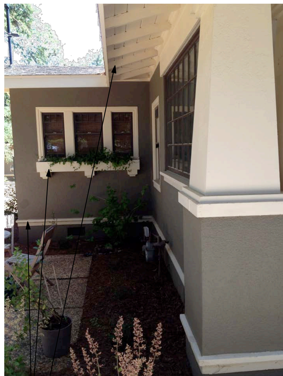
(E) PAINTED WOOD RAFTER TAILS, WINDOW TRIM, ETC.
