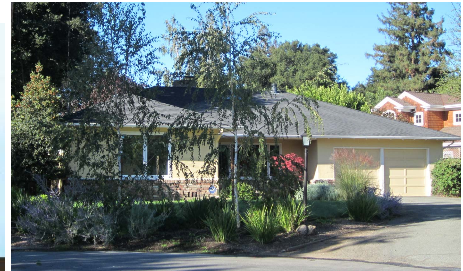
EXISTING 428 TRAVERSO CT. (PROJECT SITE)
