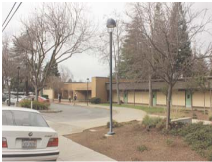
① View northwest towards Community Center main entrance
