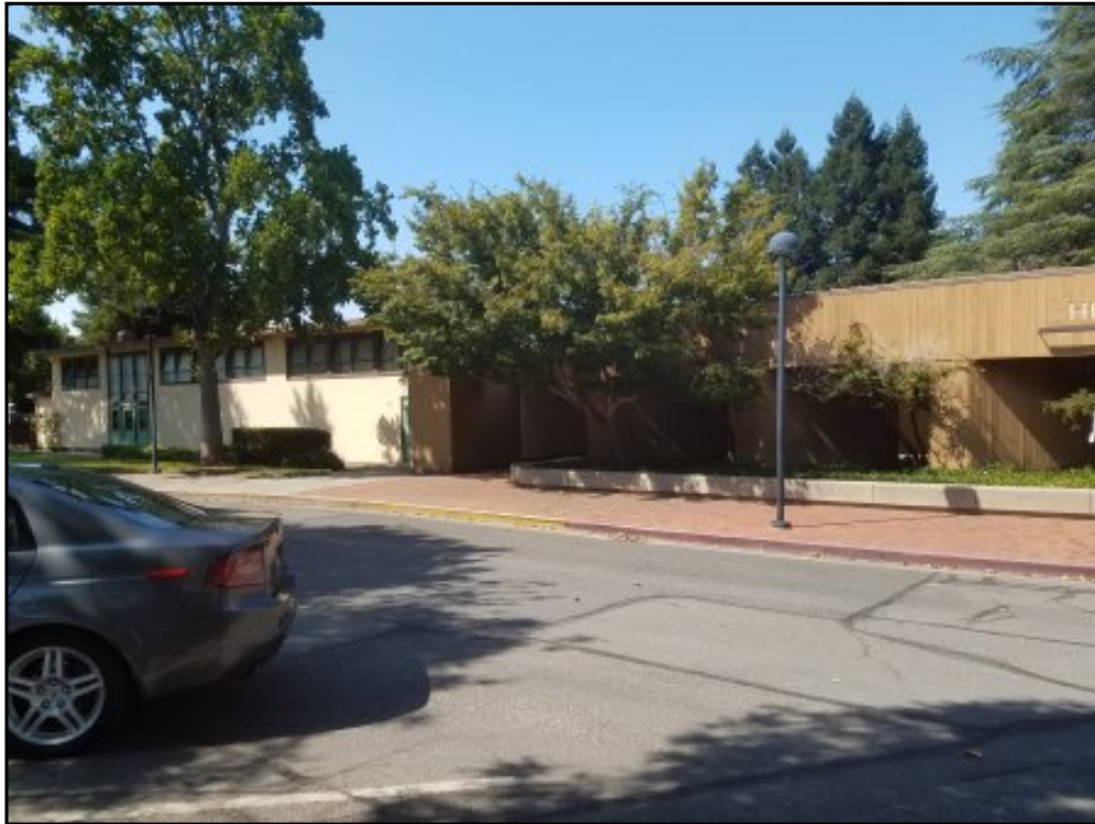
Exterior of the existing Hillview Community Center.
