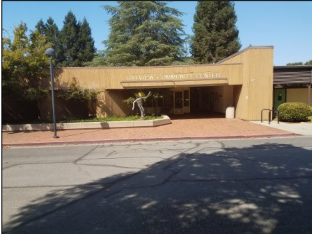
Exterior of the existing Hillview Community Center.
