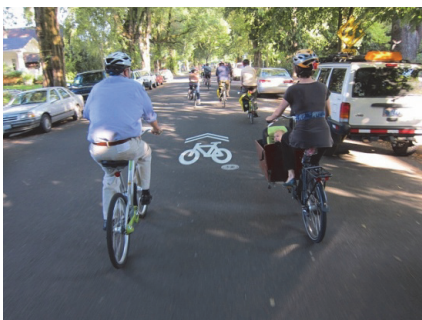
Shared Lane Markings (SLMs) delineate bicyclists' path of the travel away from opening car doors.
