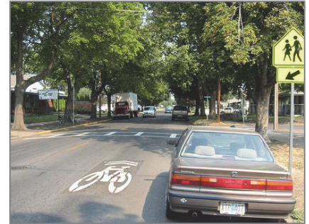
Shared Lane Markings delineate the bicyclist path away from opening car doors and inform motorists of the presence of bicyclists.
