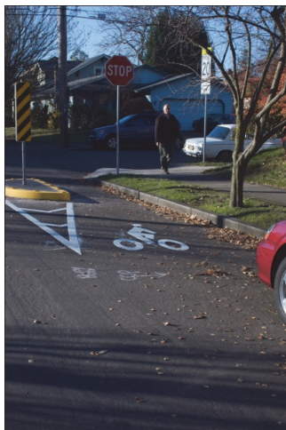
Detached curb extensions allow for “cycle slips,” or “chokers,” a design to consider when implementing the Traffic Calming Master Plan.
