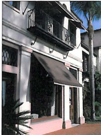
The upper and lower facades of this building work as one unified structure.
