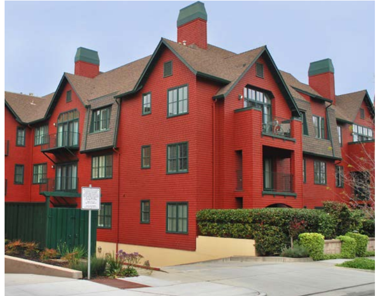
Existing three-story, standalone residential on 2nd Street.
